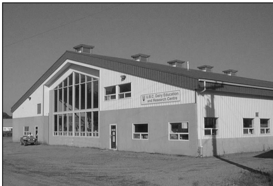
The UBC Dairy Centre at Agassiz
