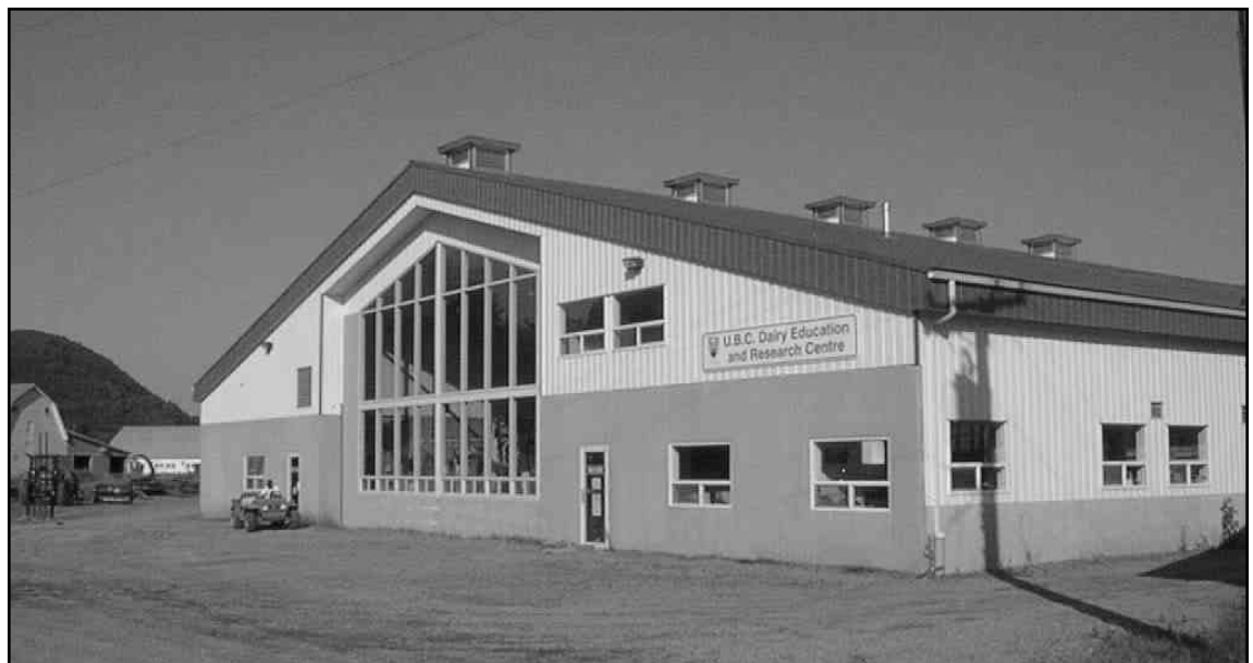
The UBC Dairy Centre at Agassiz.
